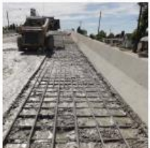
Hydrodemolition Bridge Rehabilitation
