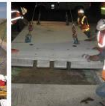
Precast Concrete Pavement Panels
